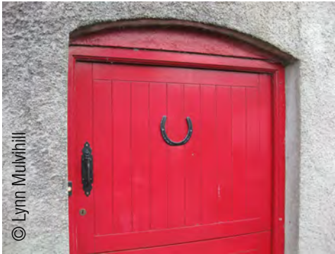
Half-door at the Old Grain Store cottages in St. Mullins
