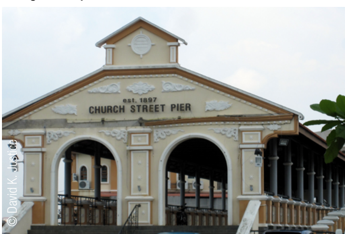
Church Street Pier at Weld Quay
