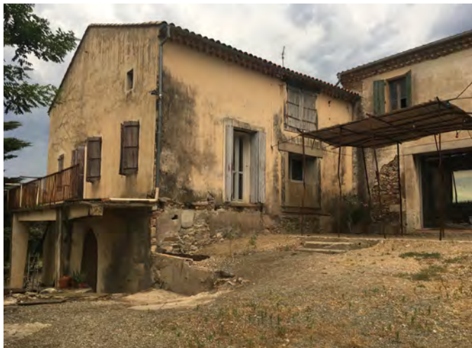
Old farm houses are a great renovation project...
