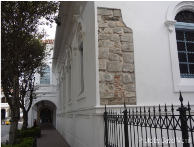
Inca stones from Pumapungo were used to build this El Centro church
