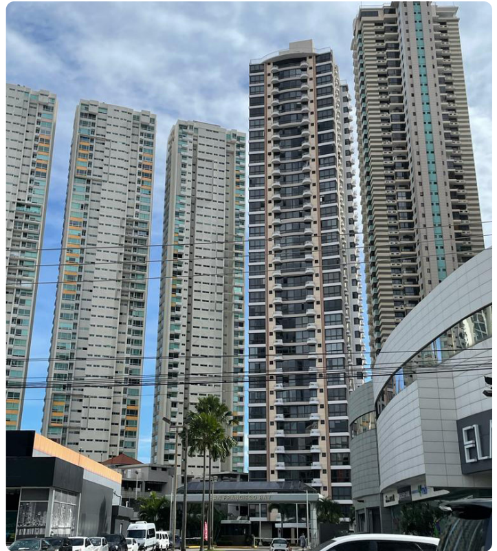
The San Francisco Bay apartments offer stunning sea views and easy access to the Corredor Sur
