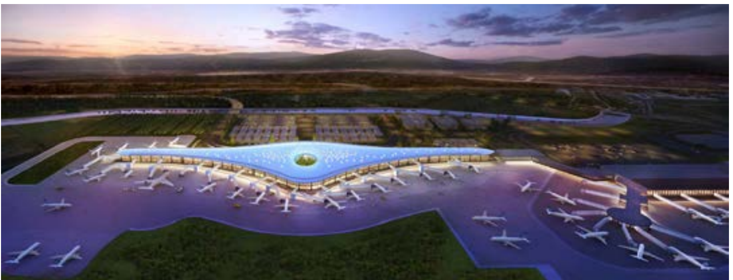
Tocumen's T2 terminal is expected to open sometime next year
