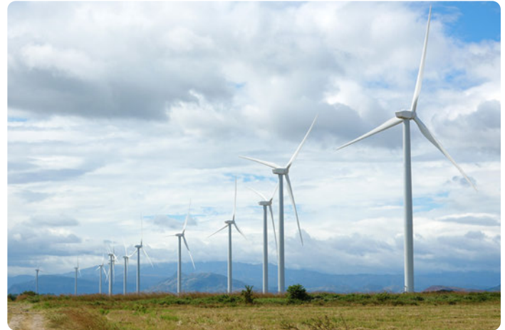
Penonomé Wind Farm Project
