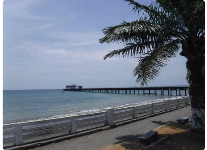
Puerto Armuelles pier
