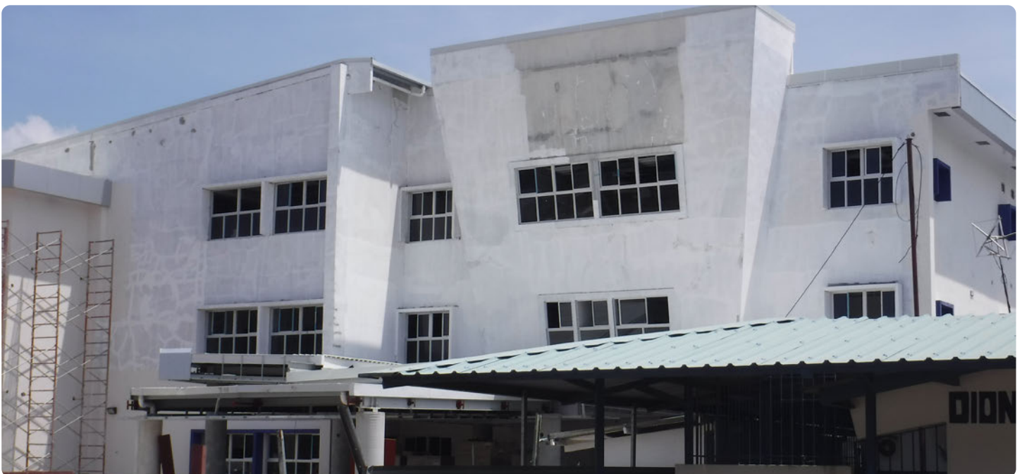
Hospital Dionisio Arrocha under renovation
