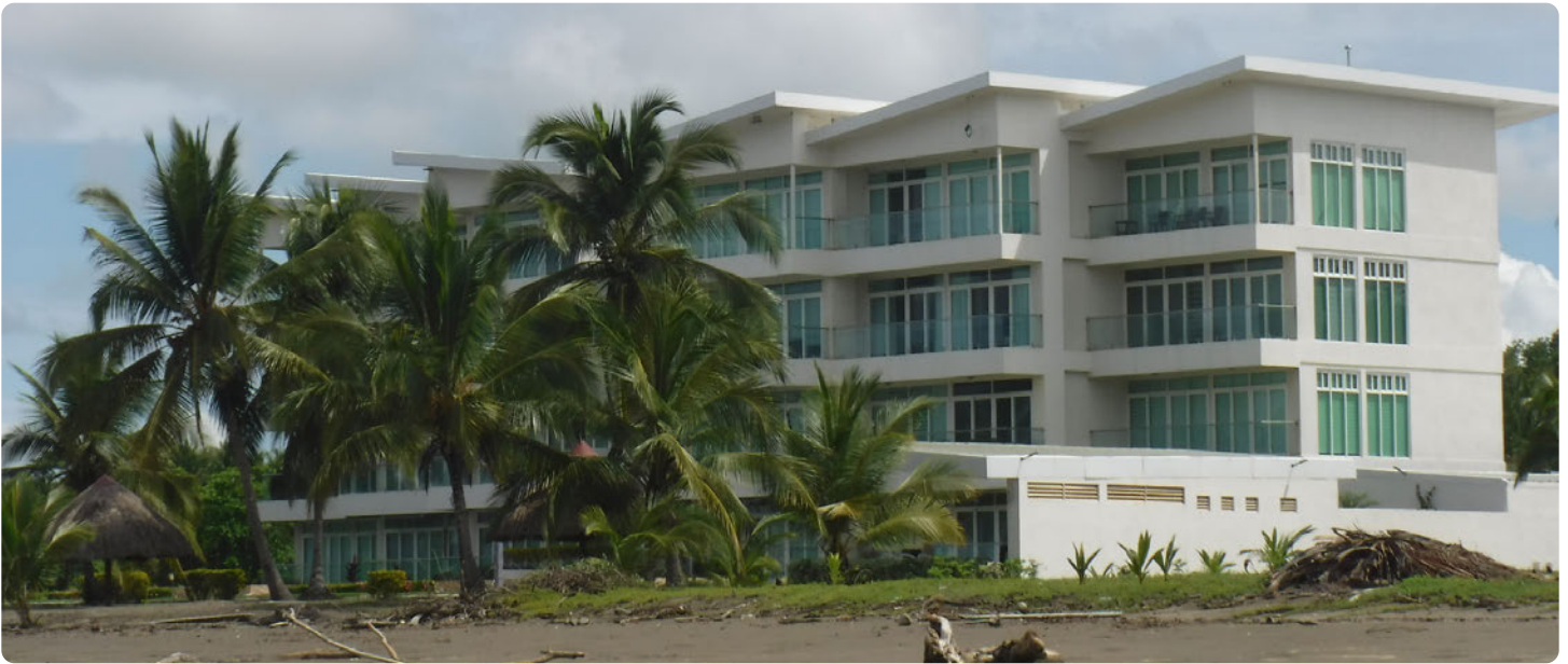
The sole condo building in Las Lajas
